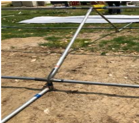
Leg poles on ground, ready for assembly after tarp is put on:
