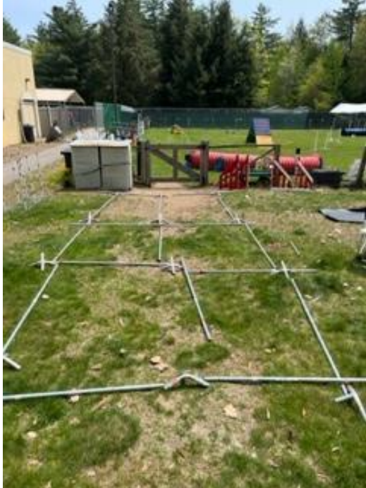
Roof parts laid out and ready for assembly:
